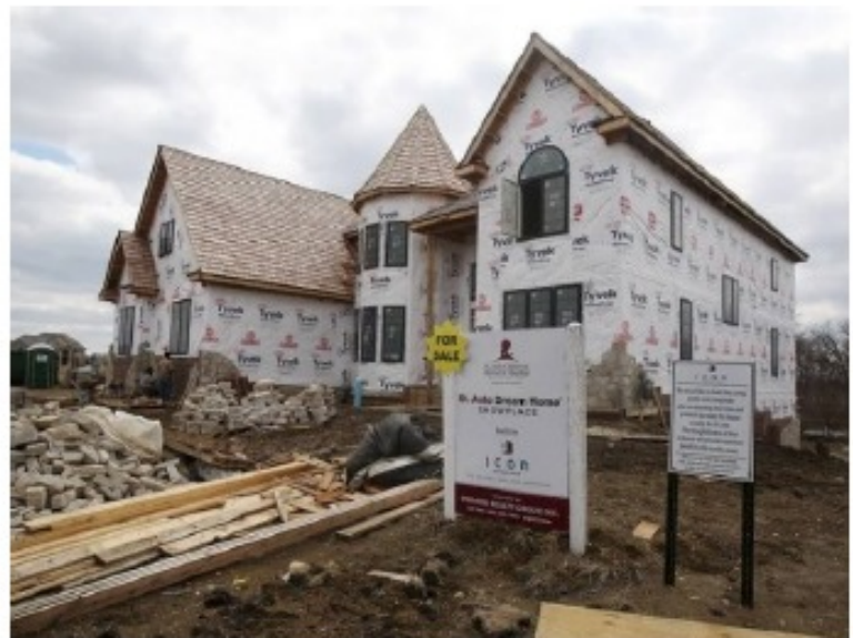
Construction crews work on a house in Vernon Hills' Gregg's Landing subdivision that will be sold to raise money for St. Jude Children's Research Hospital.
