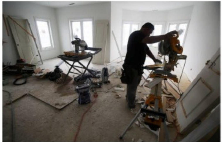
Carpenter Uriel Castaneda of Zavala's Trim Work, Inc. cuts a piece for a door frame as he works on a home in Vernon Hills that will be sold to raise money for St. Jude Children's Research Hospital. The house will have a selling price of $1.2 million and is expected to generate a donation of as much as $500,000 for St. Jude.
