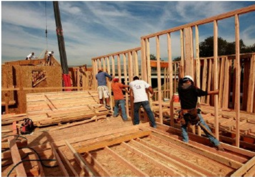
Construction workers build the frame of a house at a new housing development in Hayward, California. (Justin Sullivan / Getty Images)
